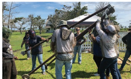
(Top) Students in UNCG’s interior architecture summer field school repaired and cleaned gravestones at Graves Cemetery on Portsmouth Island in May. (Bottom) The students worked with a mechanical tripod to suspend a gravestone, and students examined a church building’s foundation.
