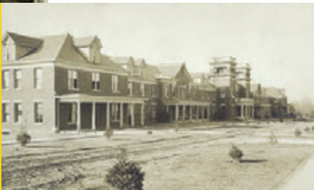
1915 North Spencer Residence Hall
